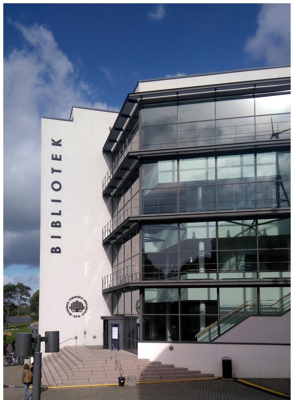
BTH library building | Photo by Martin Pekár
